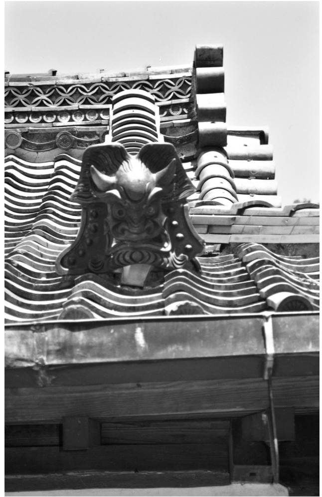
View of the Momochi house roof. Private collection.
