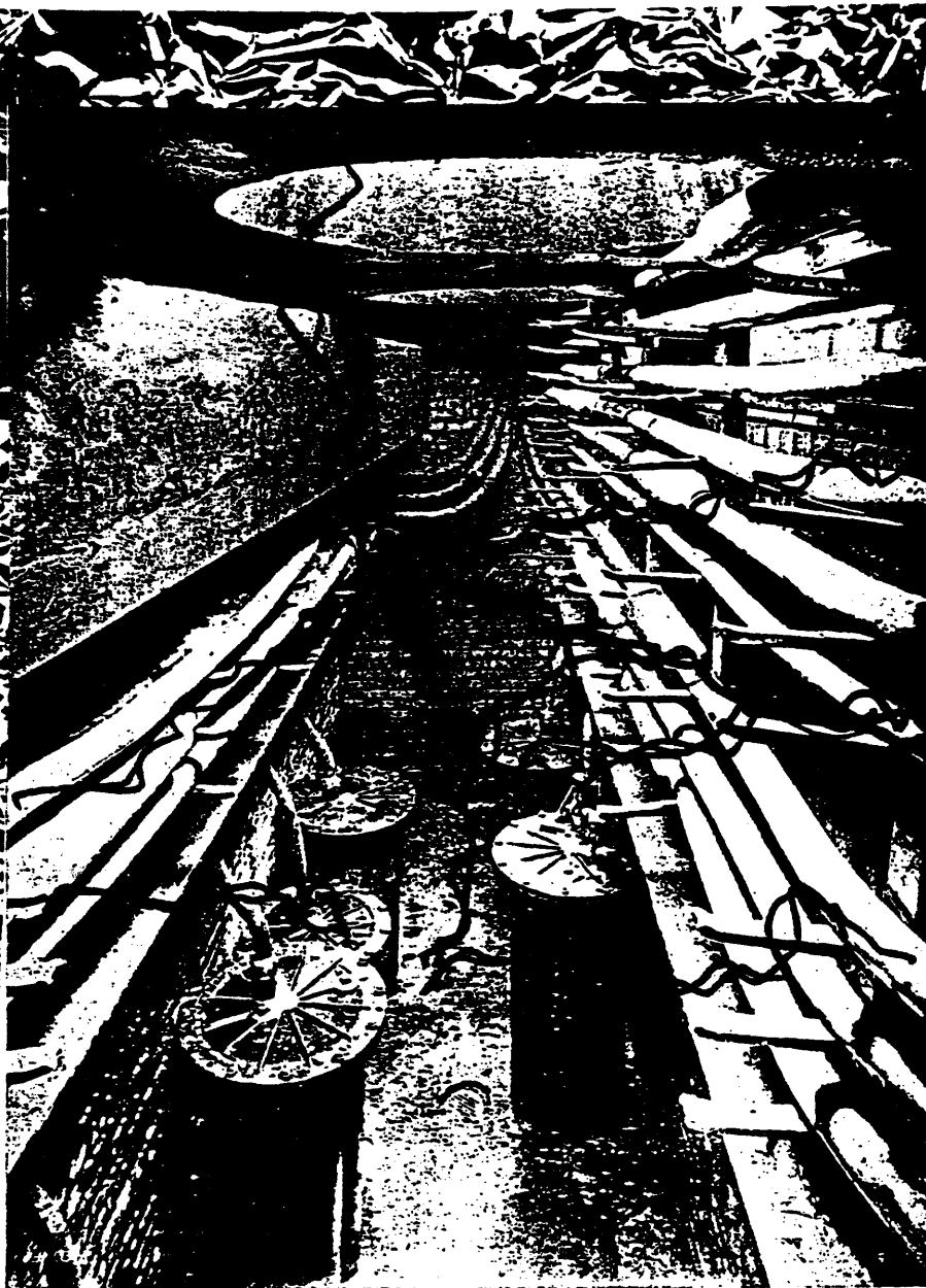
FIG. 26—Loading coil cases in a manhole, showing method of connection to cables.
