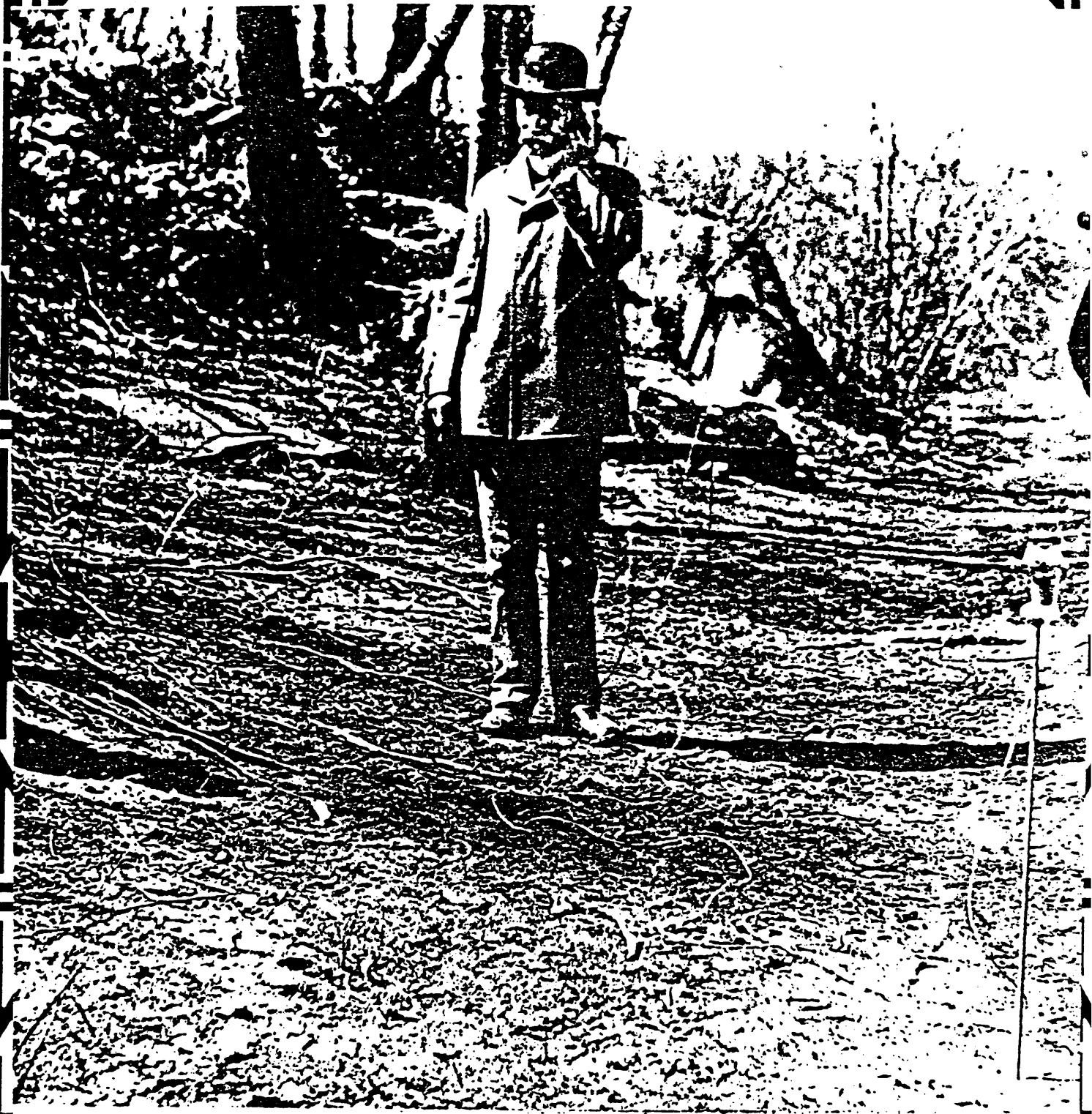
Nathan Stubblefield, \frac{3}{4} of a mile from Central Office, receiving messages by Wireless Telephone. Note the two steel rods in the ground, which establish connection with the electrical currents of the earth, being connected by 30 feet of wire attached to the receiver.
